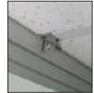
T-Grid Ceiling Attachment
